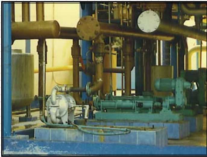
Solution providing AODD pump installation selected to reduce total costs of ownership and minimize floor space allocation.
