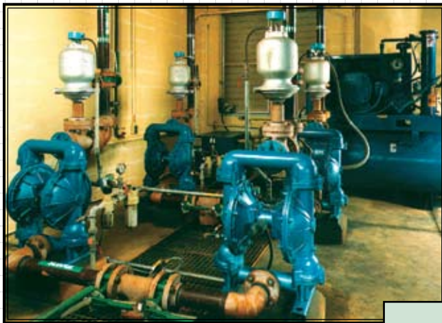
Permanently installed metallic standard duty pumps in an interior chemical industry sumping installation.
